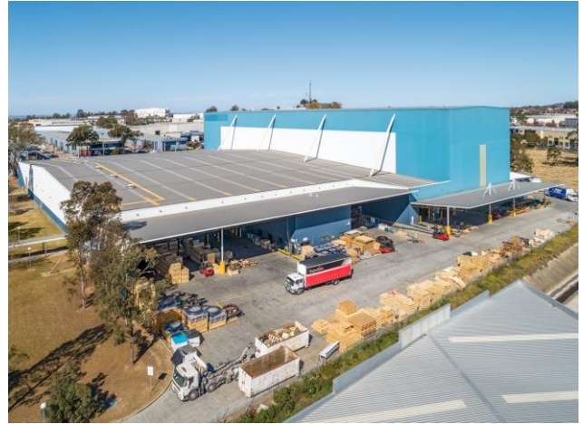
Picture 2 View of existing warehouse from the north of the site
